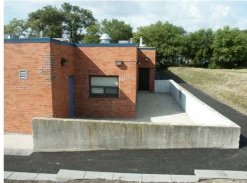
The design of the building and slope of the land has necessitated the development of a large, concrete, retaining wall in the north-east corner of the property. The retaining wall was intended to serve two main functions. First, it carves out the space needed to accommodate two fire exits found at the rear of the property while providing room for snow storage. Second, it serves as its own safety barrier by acting as a knee wall for people using the path above.
